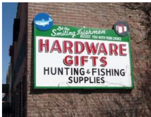
Figure 8. Acceptable fire wall sign example.
